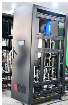
Cooling Distribution Units
